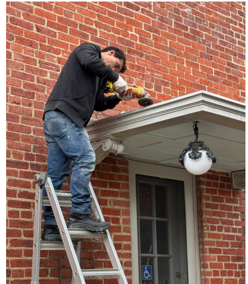
Repairing the leaking side roof
