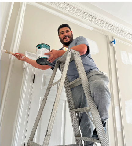
Dining Room repainting in progress
