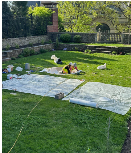
Resealing the fountain basin to prevent leaking
