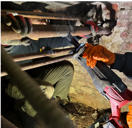
Cutting and capping failing pipes to prevent further damage
